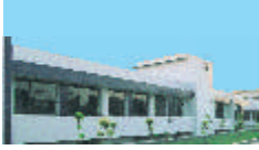
Roto's Manufacturing Plant
